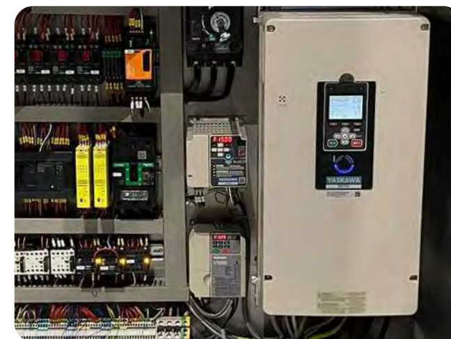
Soft start and stop of knives and bowl by mean of speed drives.
